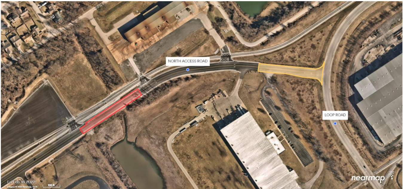
Figure 3 – Detail of North Access Road Resurfacing
